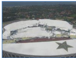
The roof collapsed on the grandstand. — Picture courtesy of PWD
