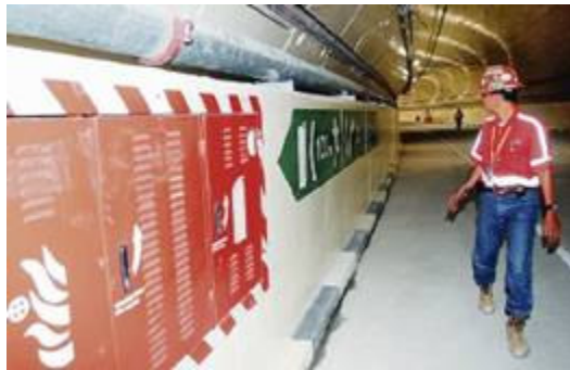
A safety worker checking emergency equipment inside the Smart tunnel. The tunnel is used to transport vehicles and drain away excess floodwaters which are stored in holding ponds
